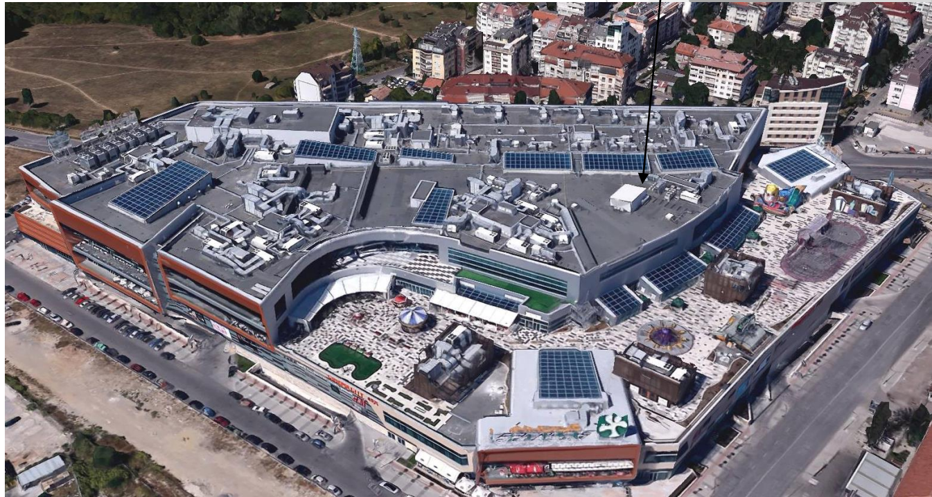
PARADISE CENTER, SOFIA, BULGARIA THE BIGGEST SHOPPING MALL IN EUROPE WITHOUT EXPANSION JOINTS WITH LENGTH = 315 M
