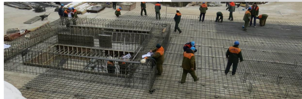
FOUNDATION SLAB REINFORCEMENT
