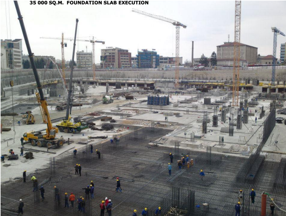
35 000 SQ.M. FOUNDATION SLAB EXECUTION
